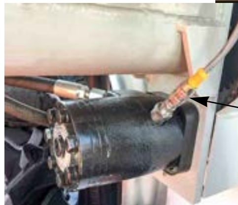
Sensor cable connected
